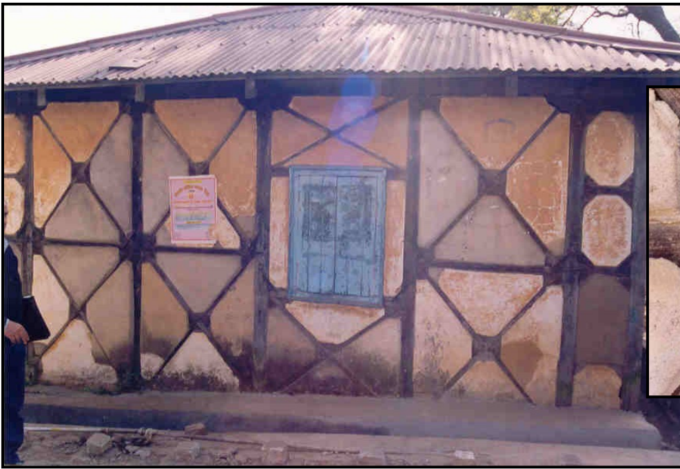
Picture 9: Dhajji-diwari building in Dharamsala. This was built after the 1905 Kangra earthquake by the British colonial administration. The diagonal bracing is effective in absorbing shear and tension forces.
