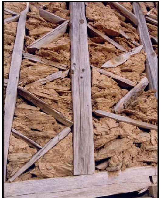
Picture 11. Detail of dhajji-diwari in Mandi district. Notice the loose mud masonry and plaster, which will absorb shocks during an earthquake.
