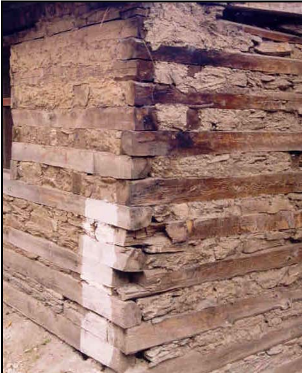
Picture 2. Corner construction detail of kath-ki-kuni style housing. The timber bands run along both sides of the wall and are connected by pins along their length, and at the corners.
