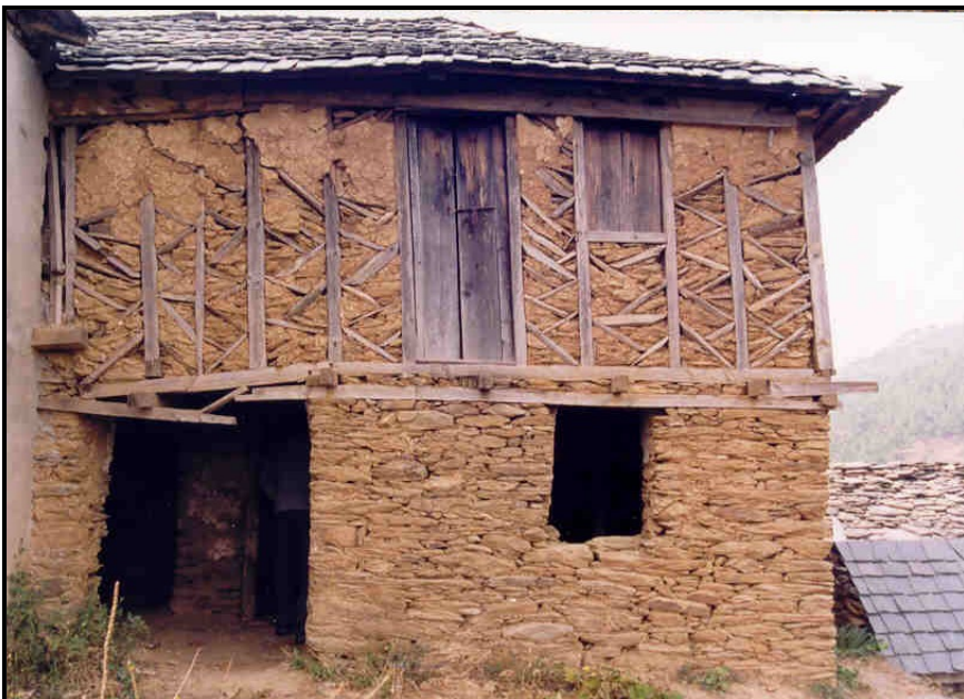
Picture 10. Dhajji-diwari construction in Mandi district of Himachal Pradesh. The pattern of diagonal bracing here parallels traditional architecture in Kashmir.
