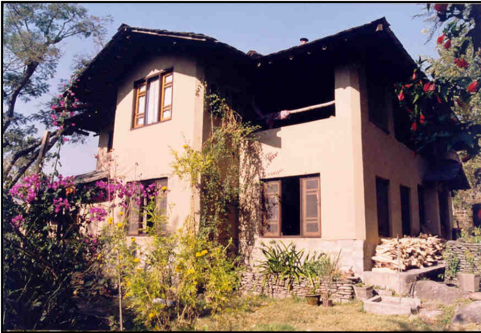
Picture 12. A house by Didi contractor in Rakkad village (Sidhbari), near Dharamsala. This house is built both with traditional materials like mud, bamboo, stone and also new materials like reinforced cement and ferrocement.
